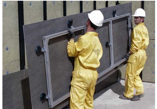
Image 7: Slab handling with Suction Frame
